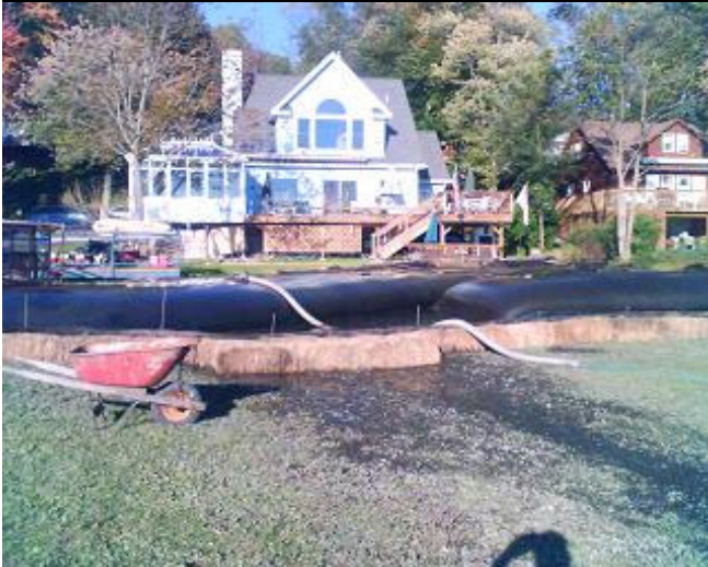
Dewatering Bags hold silt while water drains out
